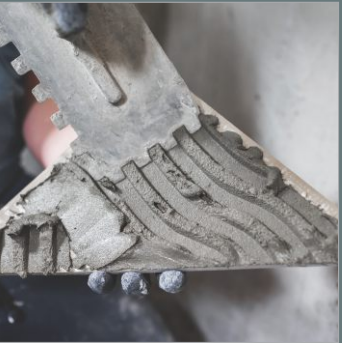
Cement laying on tile
