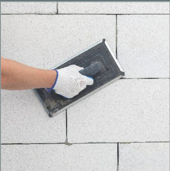
Joint Grouting
