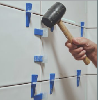
Remove wedges once it is dry
