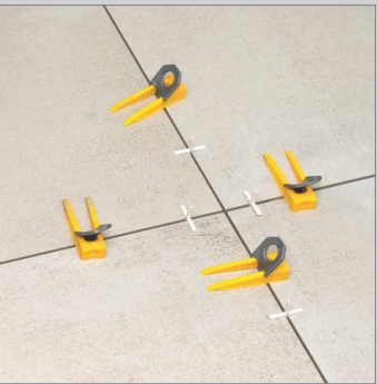
After Lavelling Process Leave Int For 8-10 Hrs.
