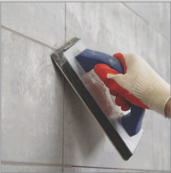
Joint Grouting
