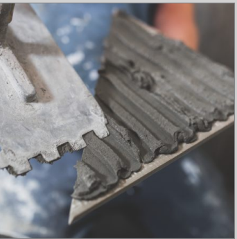
Cement Laying On Tile
