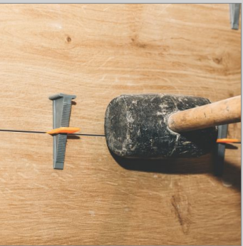
Remove Wedges Ones It Dry
